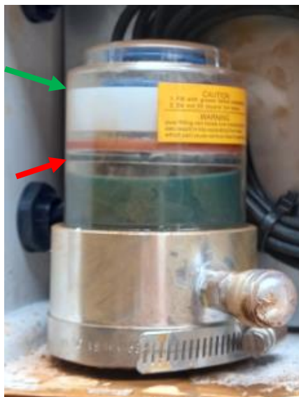
SAPO Seal Accumulator at normal fill level, with top of piston (indicated green) and bottom of piston (indicated red)
